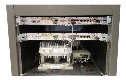
The microwave link guarantees synchronization of multiple TV transmitters with overlapping coverage area to ensure operation without mutual interference.
