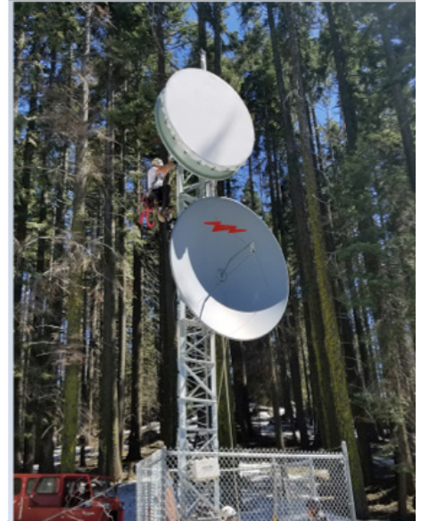
Microwave System Installation
