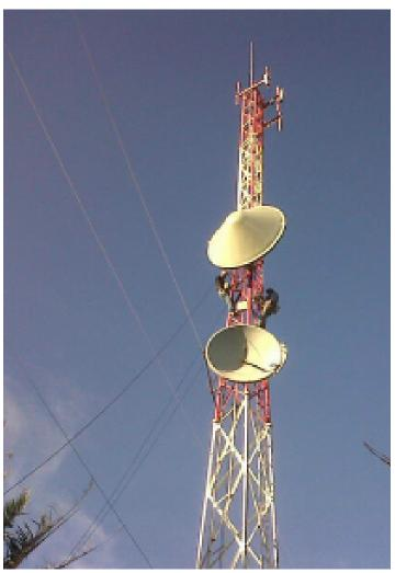
Cable Color performed the installation and commissioning of the link, including the mounting of 2,4 meter diameter antennas at a tower height of approximately 80 meters.
