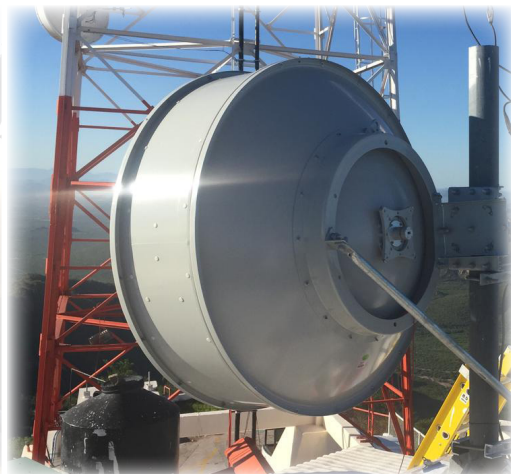
Installation of receiver antenna
