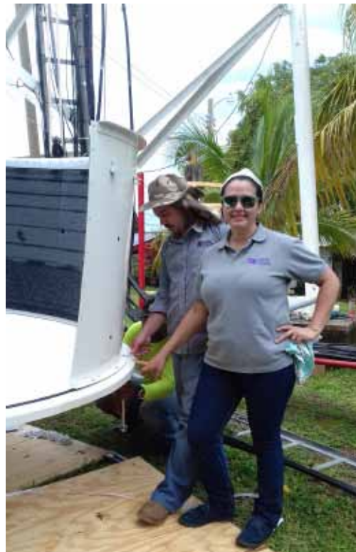
Cable Color Operations Manager, Eng. Wendy Romaña, installing IP Link
