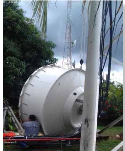
2.4 Meter Antenna Installation
