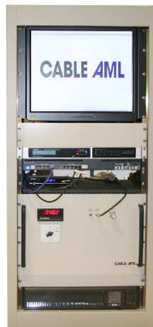
DVB-C Transmitter Station
