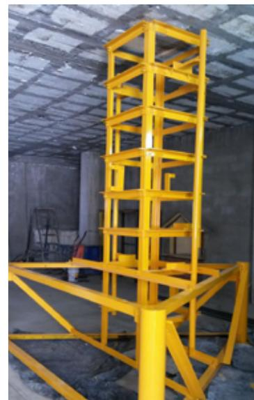
*Turret structure to mount the UHF panel antennas*
