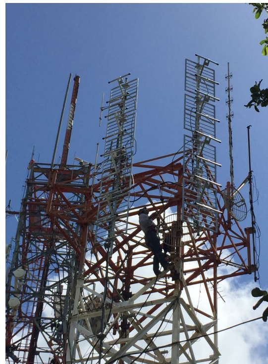
ABS personnel installing antennas.
