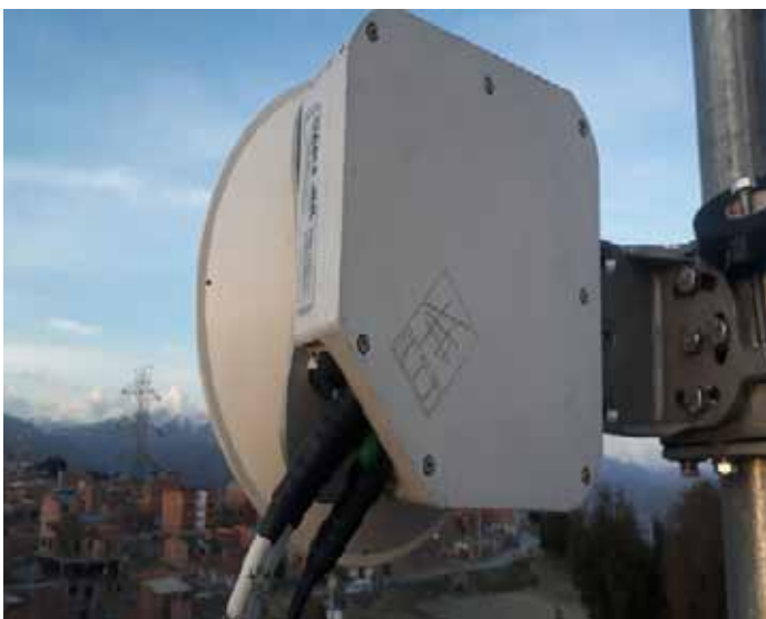
CPE (customer terminal) installation
