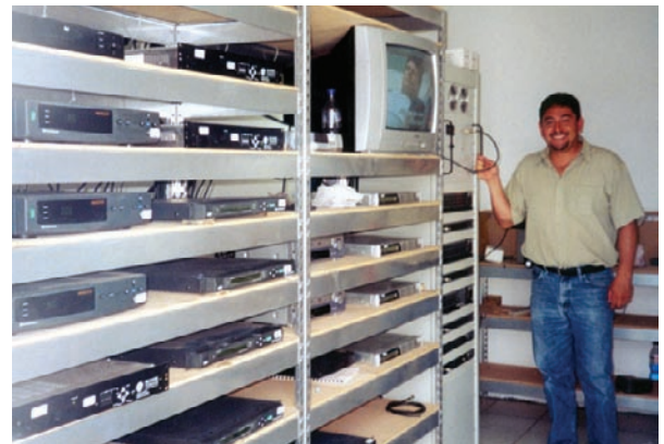
Armando Carrillo inspects the newly installed MMDS transmitter in Zacatecas
