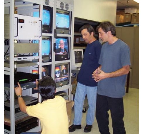
Steve and Mark Mouradian of Armenian World TV inspecting the Digital MMDS equipment at Cable AML prior to delivery.
